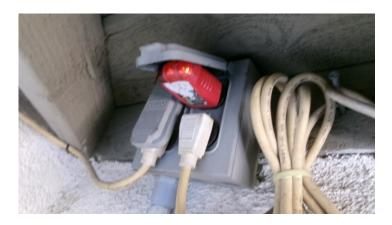
**2.** Improperly fitted light at the above location should be fitter to wall and caulked to prevent water and pest intrusion.
