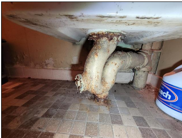
Mechanical Closet (basement)
