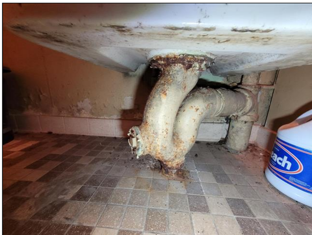
Mechanical Closet (basement)
