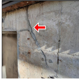
5.3 Item 2(Picture) A view of the failed crack repair at the basement foundation wall
