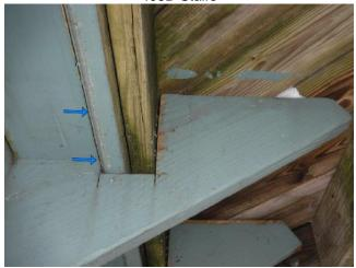
The stringer connection to deck is not properly supported. This is poorly supported with minimal support.
