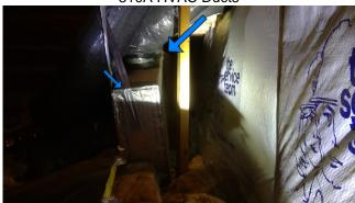
Section of separated duct work / improperly supported
