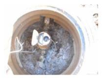
Location of main water supply valve: Valve is located at the water meter.
