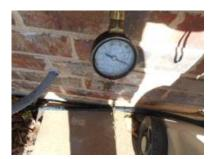
The water meter drip indicator showed no signs of flow to the structure when no demand was called for at the structure. Kitchen, bathroom, and exterior fixtures were operated. Municipal service is primary water source. SUPPLY PIPING TYPE- Piping, where visable, is copper.
