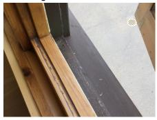
Evidence of moisture damage was observed at the rear bedroom sitting room windows. The extent or cause of damage cannot be determined without destructive analysis. Hidden damage may exist within inaccessible areas. We recommend review by a qualified, licensed contractor to locate and correct the moisture source and for necessary maintenance and/or repairs to any damaged materials, prior to close of escrow.
