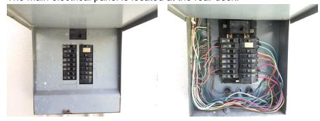
Branch circuit wiring is copper
