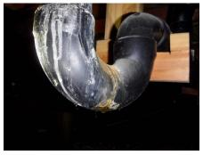
Improperly installed sanitary tee directional drain fitting(s) noted in a number of locations at the hallway bathroom. Recommend review by a qualified, licensed plumber for repair or replacement, as necessary.
