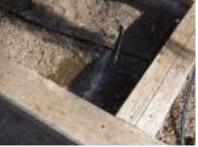
(3) Low pressure noted at left front grass area in back yard, possible broken pipe. Suggest repair/replacement as needed.
