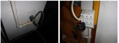
Ground fault interrupter (GFCI) provided for safety. The outlet(s) were tested, tripped and operational at time of inspection.
