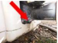
This pool system is equipped with a Chlorine Generator. During electrolysis, salty water is forced across a special metal cell that is charged with a electrical current. This process creates chlorine.
