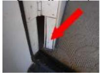
(2) Door at off of Master Bedroom opens/swings to the outside, suggest installing security hinges
