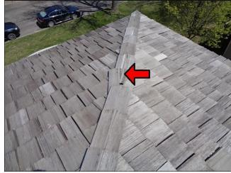
Apparent hail damage was noted. We recommend review by the appropriate insurance carriers and repair by a qualified roofer to the extent necessary to assure that the roof is both serviceable and insurable.
