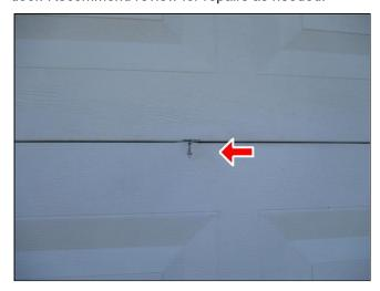
(2) Damaged weather stripping observed at the garage door. Recommend review by a qualified contractor for corrections as needed.
