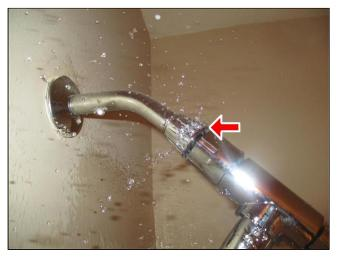
(3) The shower diverter at the shared bathroom was inoperable. Recommend review by a qualified plumber for repairs or replacement prior to close.
