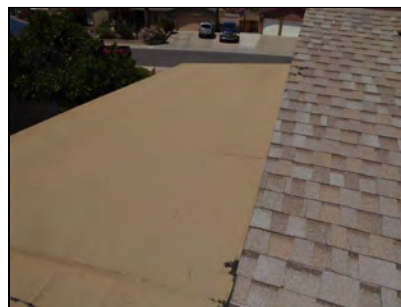
West Shed Roofing
