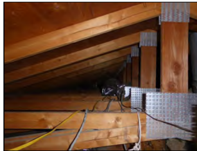
Attic - Engineered Truss System
