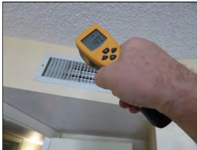
Unit 1 - Supply Air Temp
