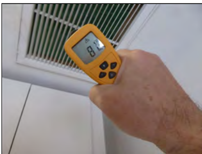
Unit 2 - Return Air Temp
