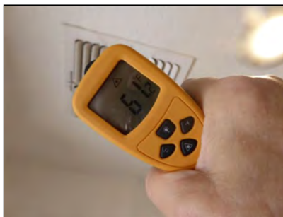
Unit 2 - Supply Air Temp
