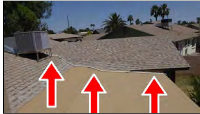
Unit 1 - Condensation Line
